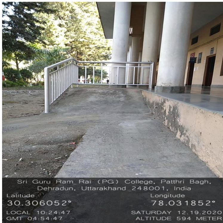
Geo tagged Photo of Ramp on Ground Floor
